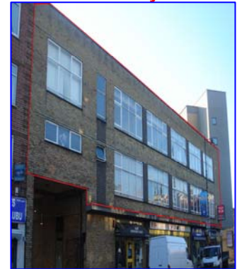
Unit 19, Celia Fiennes House, Well Street, London, E9 Second Floor Office "Let By"
