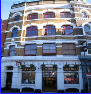
100-101 Turnmill Street, London, EC1 Office Floor "Let By"
