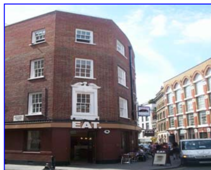
88 Cowcross Street, London EC1 Residential Building
