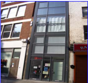
129 Whitecross Street, London EC1 Retail and Residential Building
