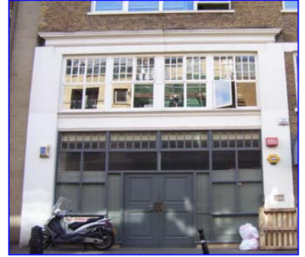
20 Britton Street, London EC1 Office Building
