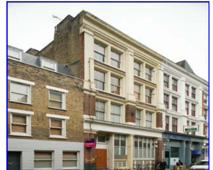
7 Mallow Street, London EC1 Residential Building
