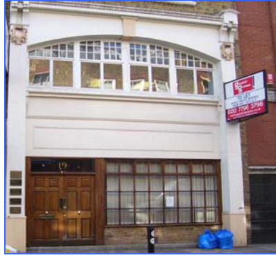
19 Britton Street, London EC1 Office Building
