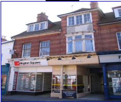
45 Winchester Street, Hampshire RG21 Retail, Office and Residential Building
